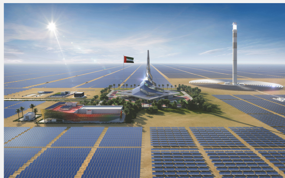
Source: Dubai commissions hydrogen plant
