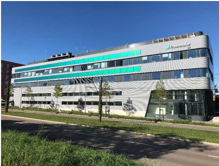
Fig.:1 Facade-integrated PV installation with green MorphoColor® panes at the Center for High-Efficiency Solar Cells at Fraunhofer ISE. © Fraunhofer ISE / Photo: Benedikt Bläsi
