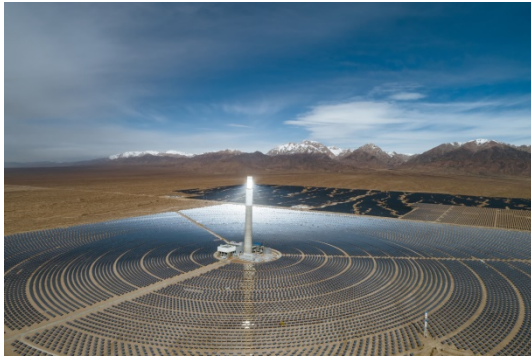
In central tower power plants, thousands of mirrors concentrate the solar radiation onto a receiver. © Shutterstock/Captain Wang
