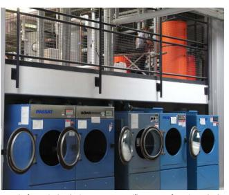
Fraunhofer ISE is developing a sector-specific concept for using solar heat in laundries, which involves solar thermal installations being integrated into the system to cover part of the heat required for individual processes. The photo above shows the storages of a solar thermal installation providing heat for boiler feed water, boiler make-up water and washing machines. ©Fraunhofer ISE
