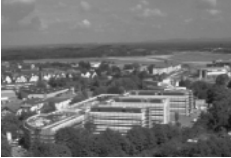
Fig. 7: New premises for Fraunhofer ISE, in autumn 2000.
