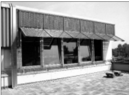
Fig. 1: PV façade system as shading for the associated training rooms.
