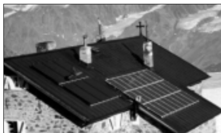
Fig. 1: Photovoltaic modules and collector field on the south-facing roof of the Brandenburger Lodge, the highest lodge of the DAV at an altitude of 3277 metres above sea-level.
