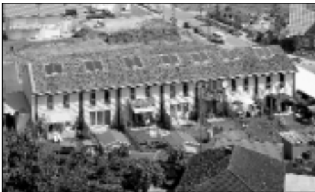
Fig. 1: View of the solar passive houses in Neuenburg.
