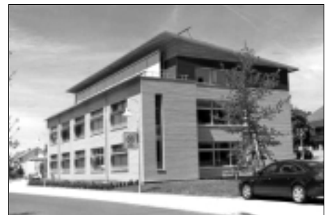
Fig. 2: The pilot study was carried out in the 10 south-facing offices of the new building for the engineering and measurement office belonging to Hans Lamparter GBR (architects: Werkgemeinschaft Maier, Weinbrenner, Single).
