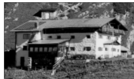
Fig. 2: Tölzer Lodge, at an altitude of 1825 metres above sea-level. The entire electricity demand is met by 35 m 2 of solar cells with a rated power of 3.5 kWp and a 750 W wind generator.
