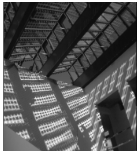
Fig. 3: A view up to the top of the atrium. The photovoltaic generator projects a shadow pattern onto the curved wall of the atrium.
