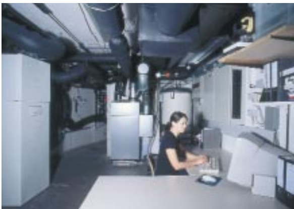
Fig. 1: Automated test facility with two testing stations to measure ventilation units and exhaust-air heat pumps.
