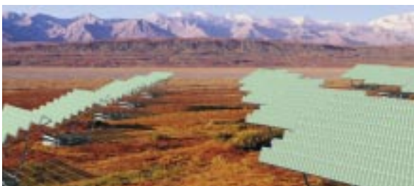
Fig. 2: Visualisation of a photovoltaic power plant consisting of many tracking units, each of which is equipped with several hundred modules.
