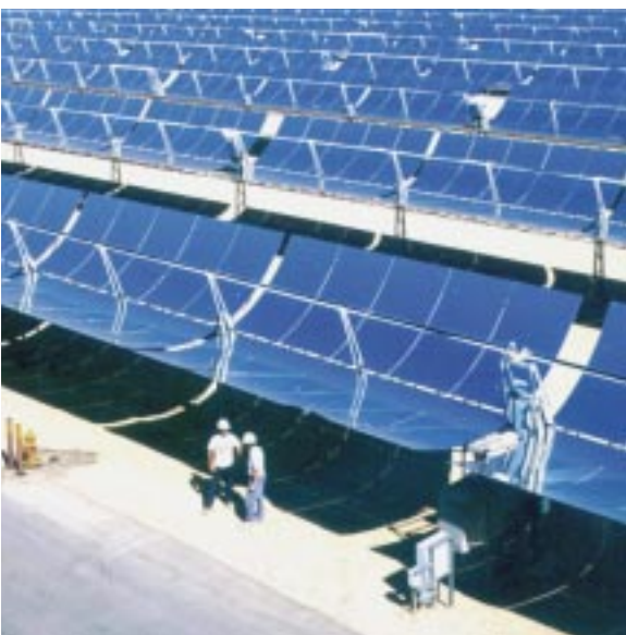
Fig. 1: Solar thermal power plant based on parabolic trough collectors in California. Parabolic trough power plants with a total electric power of 354 MW have been installed there and have proven their commercial maturity with more than 15 years of continuous operation. (Source: US Department of Energy).
