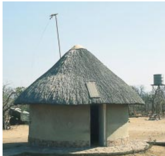
Fig. 2: Hut in an African village powered by a Solar Home System.
