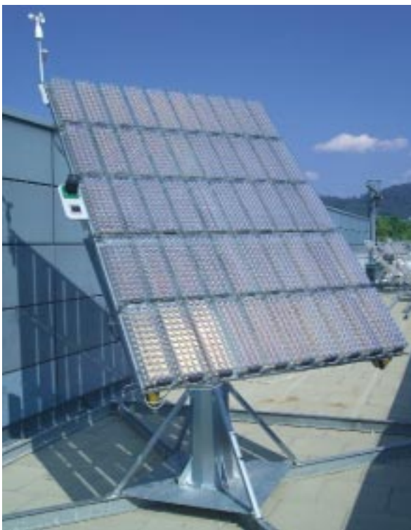
Fig. 1: Photovoltaic concentrator system with 50 FLATCON® modules on a tracker. The optimised controls guarantee tracking accuracy of 0.1°. The system feeds the generated electricity into the grid. The system shown here is located on the roof of Fraunhofer ISE.
