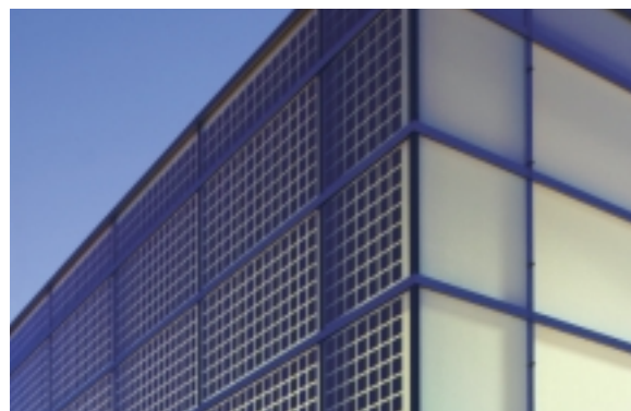
Fig. 3: Facade-integrated photovoltaics in a gymnasium in Burgweinting. Fraunhofer ISE is supporting the planning process and quality assurance during construction by integrated planning of the indoor climate and daylighting.
