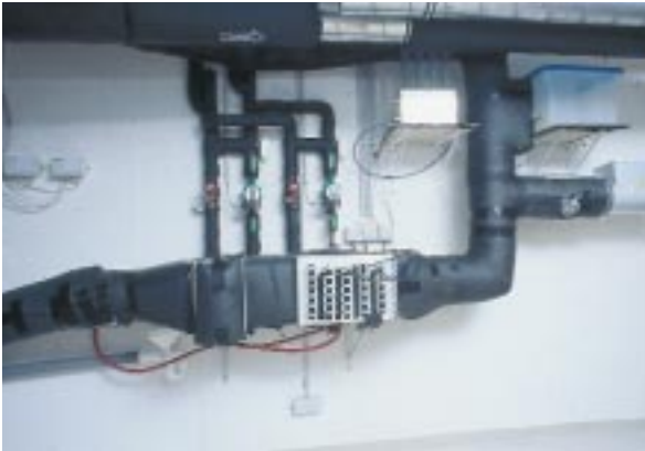
Fig. 2: Conditioning unit for outdoor air (insulation partly removed): The outdoor air flows in from the lower left through the pre-cooler/dehumidifier and the low-temperature chiller, then upwards to the ultrasonic humidifier and air heater. Two air currents can be separately conditioned as supply air and as a second heat source.
