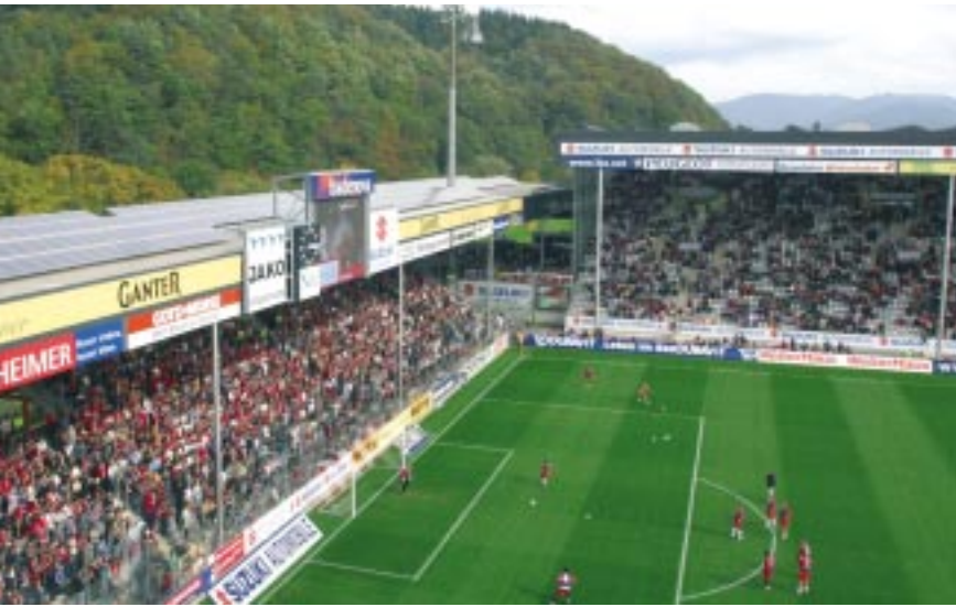
Fig. 2: The new 90 kW solar power plant on the northern tribune of the badenova Stadium in Freiburg is the first system of the 1 MW "Regiosonne" project. Here also, Fraunhofer ISE is responsible for all aspects of quality management.
