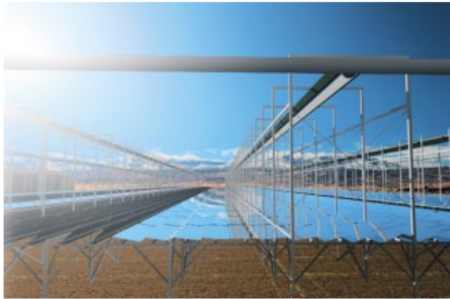
Fig. 1: Visualisation of a solar-thermal Fresnel collector array. The faceted reflector field can be seen in the horizontal plane. The reflectors track the sun individually, so that the solar radiation is concentrated onto the linear absorber tube above.
