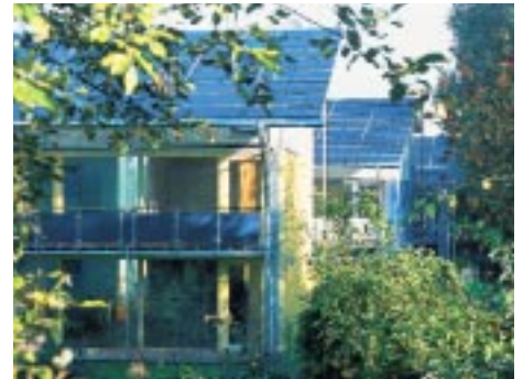
Fig. 2: In the “Solarsiedlung Schlierberg”, about 130 inverters feed electricity from about 330 \text{ kW}_p of installed photovoltaics into the low-voltage grid. Photo: Andreas Weindel
