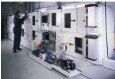
Fig. 1: The air-handling unit is the core of the test stand for desiccant cooling systems.
