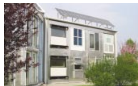
Fig. 1: Facade test facility of Fraunhofer ISE: The two lightweight cells are positioned above each other (centre of photo).
