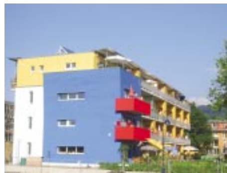
Fig. 2: Monitoring of the house belonging to the "ISIS" building co-operative began in winter 2002. Architecture: M. Hansen, Freiburg. The building facade illustrates design options for passive buildings.
