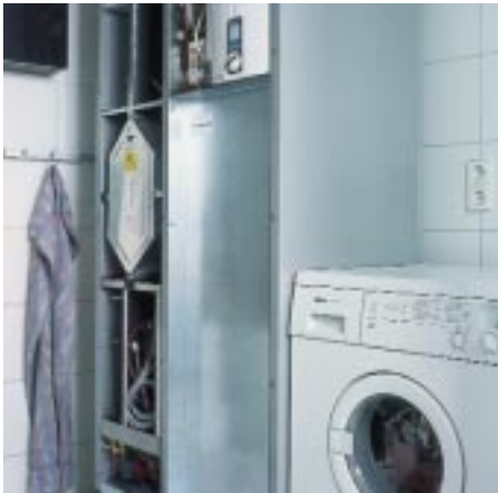
Fig. 3: The first compact ventilation and heating unit designed for a whole storey by the Maico company, being tested in the ISIS passive house as an experimental prototype with a simplified design. The compact unit is not larger than a combined refrigerator/freezer, and can be located inside the flat, e.g. in the bathroom, without occupying too much space.
