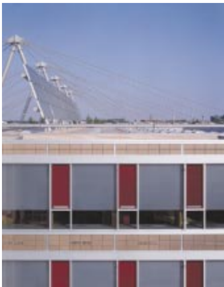
Fig. 1: Facade and roof construction of the SOLVIS zero-emission factory (Photo: C. Richters).
