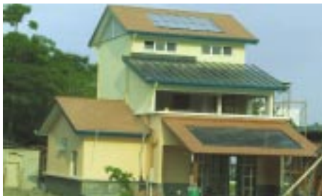
Fig. 1: View of the “solar house prototype”. Standard silicon modules are located on the upper roof, silicon thin-film modules are mounted on the middle roof and the lower roof is covered with photovoltaic polycrystalline roofing tiles.
