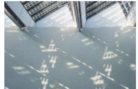
Fig. 4: Sawtooth roof with integrated photovoltaics in the atrium of the new building for Fraunhofer ISE.
