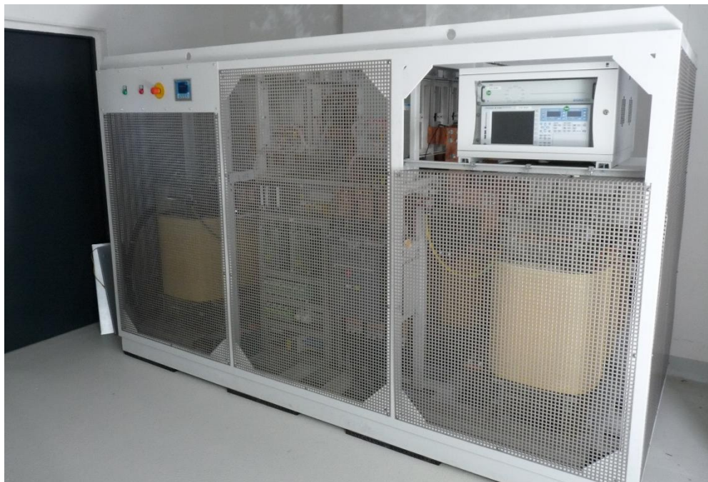
Figure 2-14: Thyristor rectifier system of a 1 MW electrolysis stack test lab at Fraunhofer ISE
