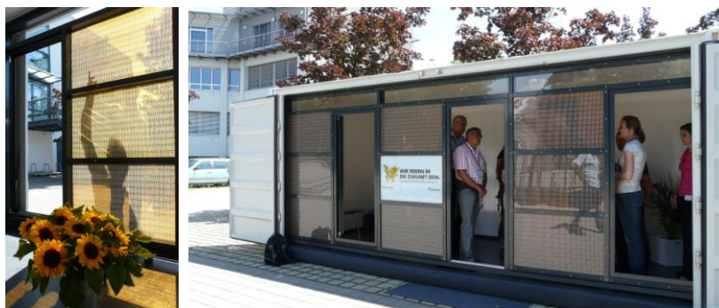
Figure 3: Dye solar module showroom for BIPV applications using large area glass frit sealed DSC modules (meander type) as developed at Fraunhofer ISE 2012
